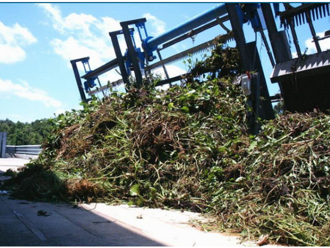
Debris effectively diverted from the pumps.
