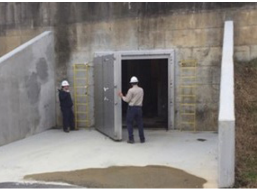
New intermediate access level door
